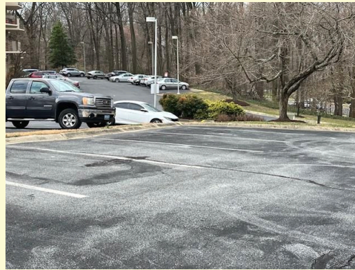
The parking spaces uphill of the sign in the picture at left will be converted to the bioretention garden.
