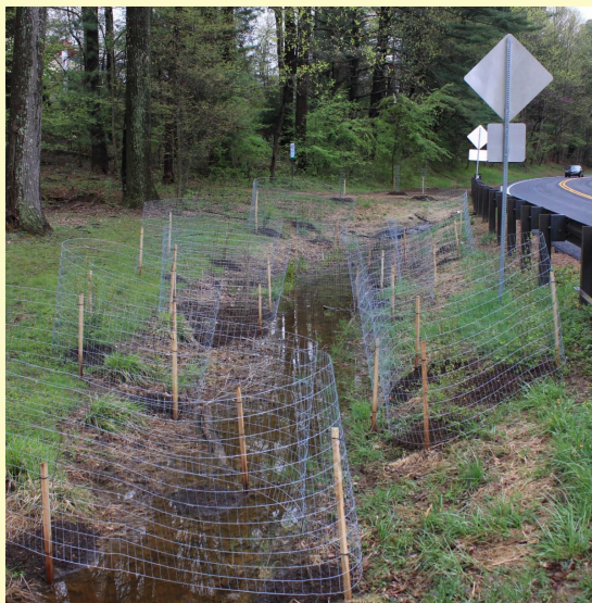
Floodplain depression planting along Sligo Creek Parkway just downstream of University Blvd. immediately after installation (above) and later that summer after herbaceous plants were added (Parks photos)
