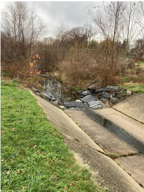
Figure 2. Concrete channel feeds directly into Evans Parkway neighborhood park.
