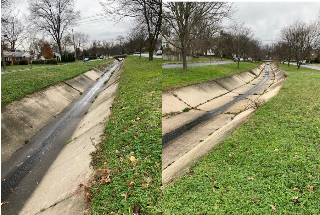
Figure 1. Concrete channel along Bucknell Drive.
