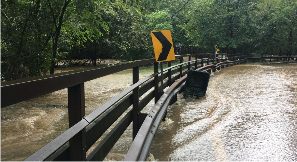
Sligo Creek and hiker-biker trail (left) and Parkway (right) just upstream from the Maple Avenue bridge following massive rainstorm on September 10 (Naomi Edelson photo)
