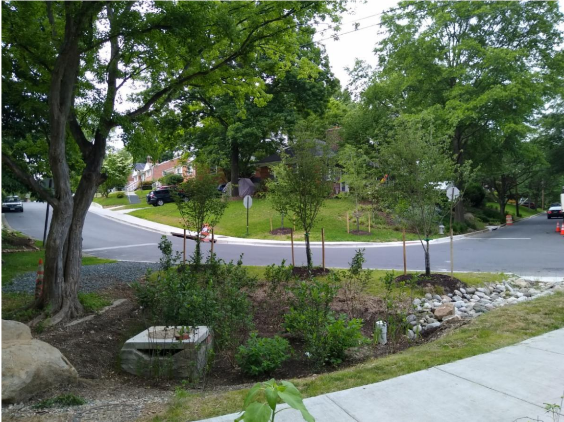
This rain garden at Jackson is designed to collect stormwater from flow off the street surface from the input lined with stones at right.
