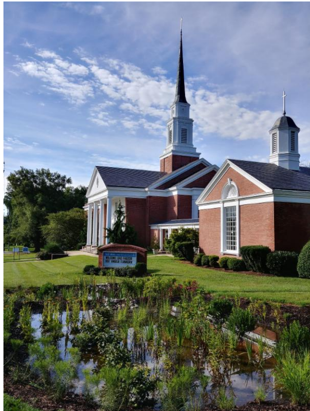
New rain garden at Silver Spring United Methodist Church on Georgia Avenue
