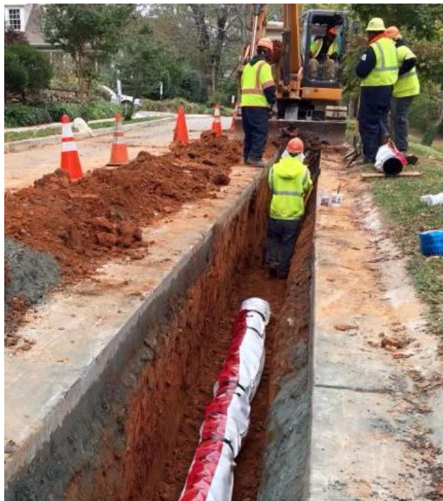
WSSC crew installing the kind of zinc-coated ductile iron pipe wrapped in protective coating that will go into the Colesville Rd project (WTOP photo)
