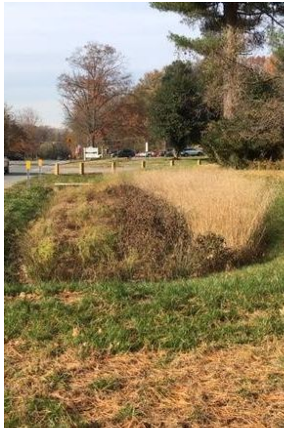
Bioswale along the Parkway at the golf course
