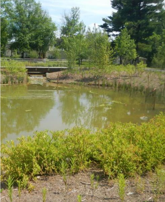
One of three new ponds, with plantings and viewing deck
