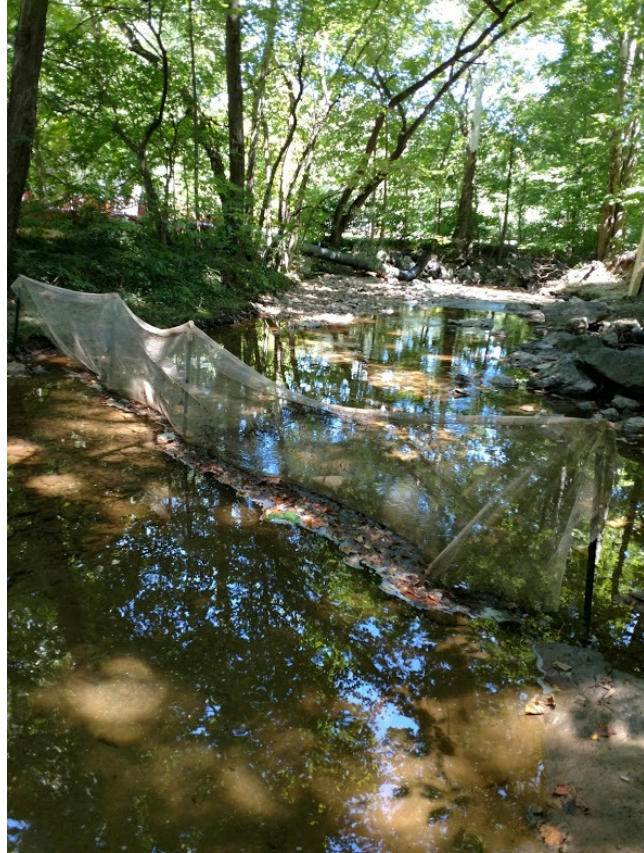
Netting across Sligo will keep fish from work areas during stream bed restoration.
