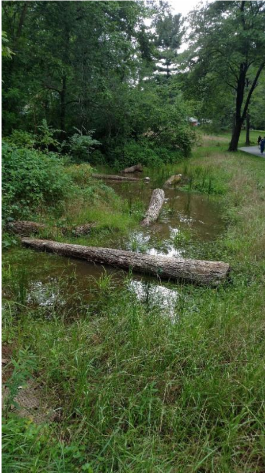
Shrubs and trees will be planted at this stormwater swale across from the south end of the soccer fields. (Wilpers photo)
