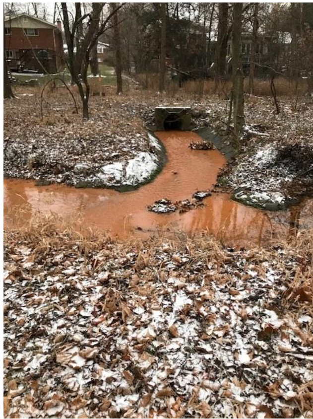
Sediment flows from water line break into Sligo Creek Park. Note clear water, far right, upstream from sewer outfall. (Murtagh photo)
