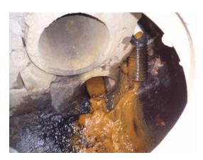
Figure 12. Four pipes enter a stomrwater manhole at Glaizewood and Devonshire. Ammonia was elevated from the flow being discharged from the black, corrugated pipe (0.25 mg/l in field, 0.14 mg/l checked with spectrophotometer later in the day).
