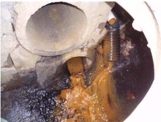
**Figure 12. Four pipes enter a stormwater manhole at Glazewood and Devonshire. Ammonia was elevated from the flow being discharged from the black, corrugated pipe (0.25 mg/l in field, 0.14 mg/l checked with spectrophotometer later in the day).**
